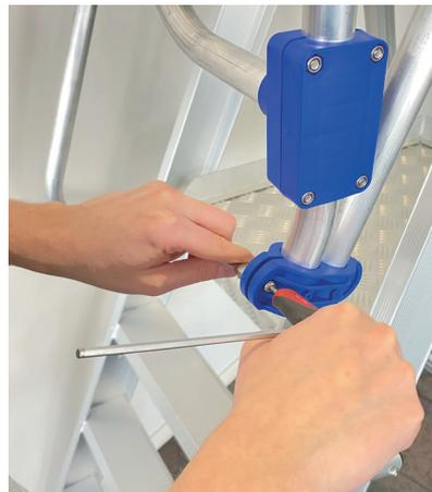
4. When both doors are in place, align them with each other. To align the clamps, align the front locking hole with the hole in the bracket.
